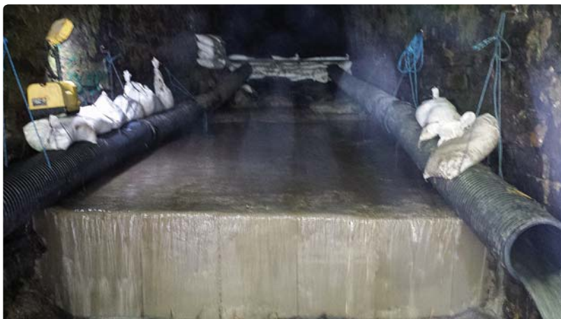
Completed concrete invert reinstatement.
