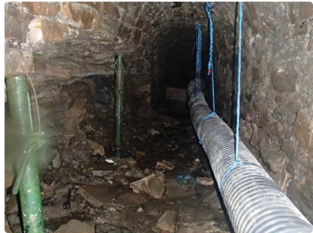
Masonry arch culvert with collapsed abutment and scoured invert, and with temporary works in place.
