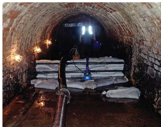
Water management temporary works in Nant Tysswg culvert.
